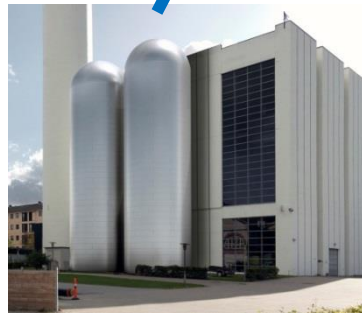
Thermal storage tanks
